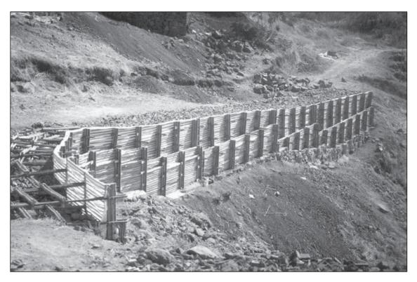
Figure 7: Bamboo retaining wall
